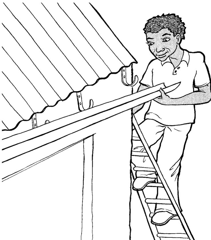
*Figure 4: Connecting a gutter system*
